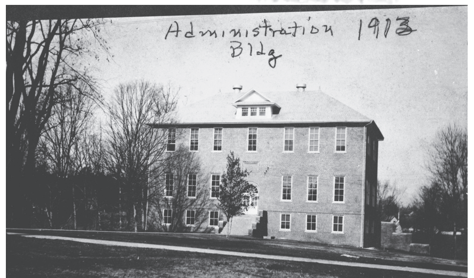
The soon-to-be-renovated Administration Building. Photo via Milligan College
